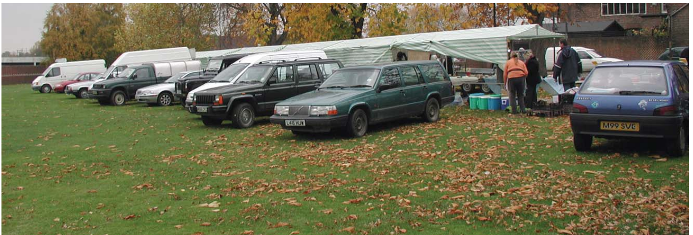
After a few months of the growing season, the grass roots have intertwined with the mesh filaments creating a strong stable surface capable of withstanding heavy pedestrian and occasional vehicular use. The grass can be cut as normal and has regained its natural appearance.
