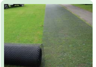
Mesh laid onto existing grassed surface
