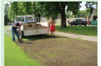
Topsoil brushed over the surface
